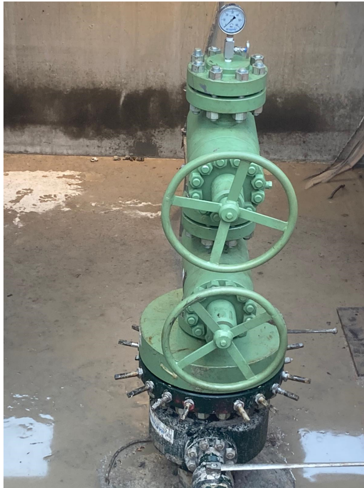
Fig. 3-13: Wellhead installed after finishing drilling operations
