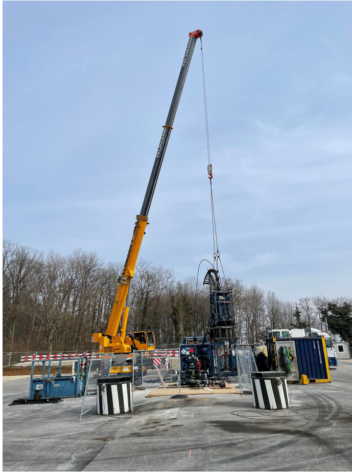
Fig. 3-14: Rigging up the coiled tubing unit from Baker Hughes
